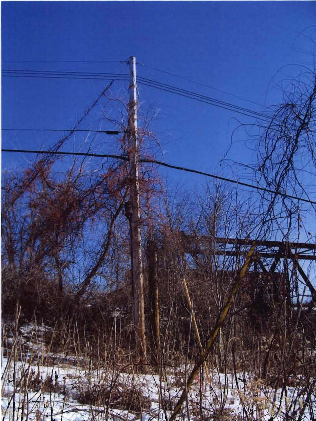
Figure 9: Concord Electric Pole 51 Note the poor vegetation management practices of the existing attachments. Note messenger or support wire at the very top of the pole is used by Concord Electric to support the covered aerial cables. Next lowest wire is covered aerial cables (aka Hendrix wires) which serves as 3 phase circuit 15H3. Next lowest cable is Fairpoint Communications attachment which dead ends at this pole. It does not span the river at this time. The lowest cable is Comcast Cable formerly MediaOne which does span the Merrimack River.
