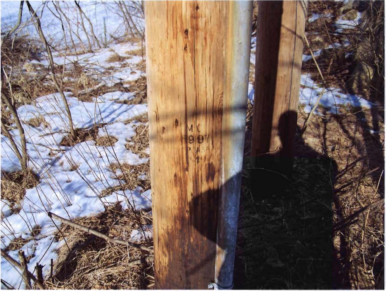
Figure 6: Concord Electric Pole #50 (southern side of Merrimack River). Note the pole to the right is the former pole that was replaced in 1998. Existing Pole height is 45 feet in length, embedded 6.5 ft into ground and is at an elevation of 235.0 ft at the bottom and elevation of 273.5 ft at the Top.
