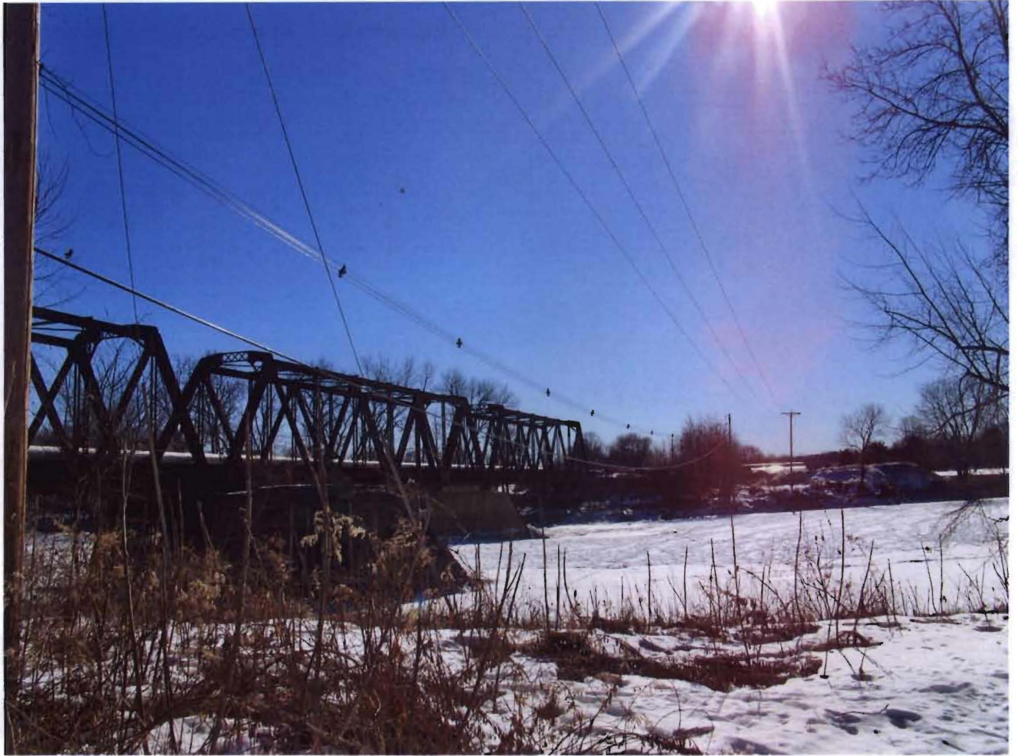
Figure 5: Looking southerly across Merrimack River, note covered aerial cable (aka Hendrix wire) used for Circuit 15H3 and lower hanging Comcast cable that is attached to Concord Electric Poles 50 and 51.
