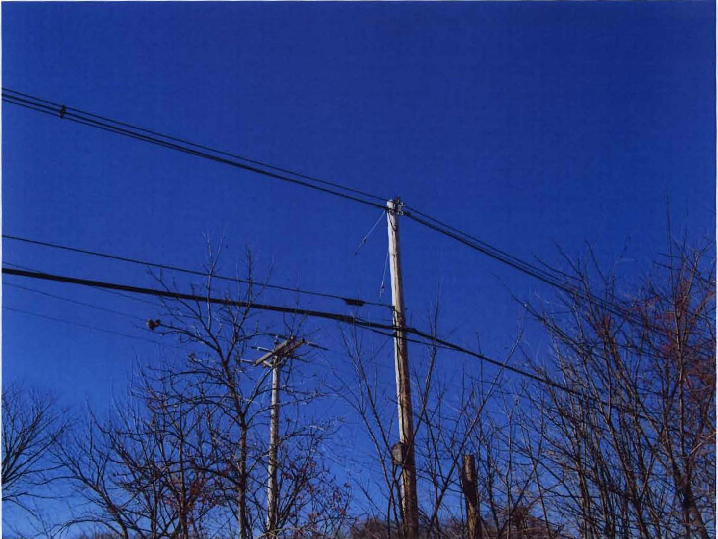
Figure 8. Concord Electric Pole 51 on the northern side of the Merrimack River Crossing. The elevation of the penetration of the pole is elev 236.9 ft and the top of the pole is at elevation 275.4 ft. Note the poor vegetation management practices of the existing attachments. Note messenger or support wire at the very top of the pole is used by Concord Electric to support the covered aerial cables. Next lowest wire is covered aerial cables (aka Hendrix wires) which serves as 3 phase circuit 15H3. Next lowest cable is Fairpoint Communications attachment which dead ends at this pole. It does not span the river at this time. The lowest cable is Comcast Cable formerly MediaOne which does span the Merrimack River.
